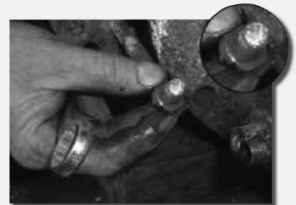
...which can lead to broken bolts.
