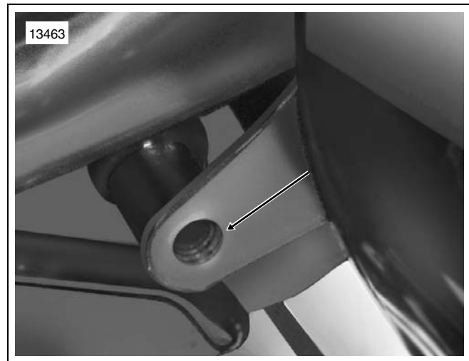
Figure 2. Front Fuel Tank Fasteners Removed
